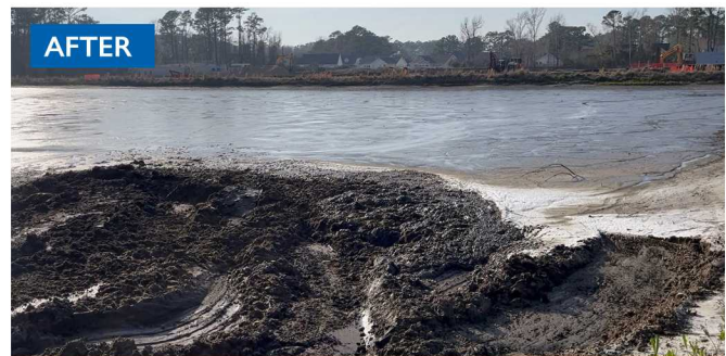
Portion of lagoon wastewater solidified with SAP.
